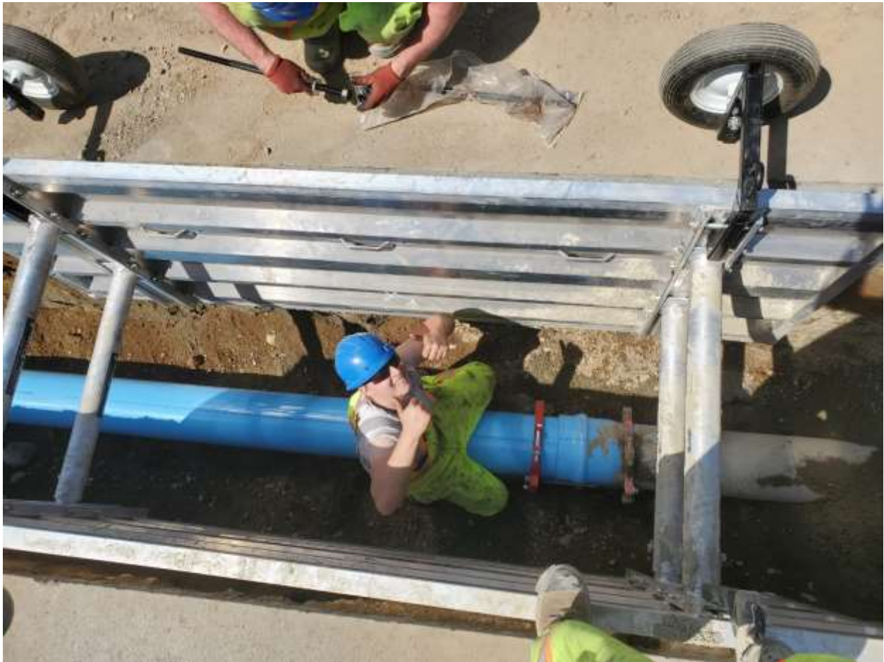
IMAGE | 2024 PIPE REPLACEMENT ALONG CONRAD AVENUE AND CARLA COURT.
