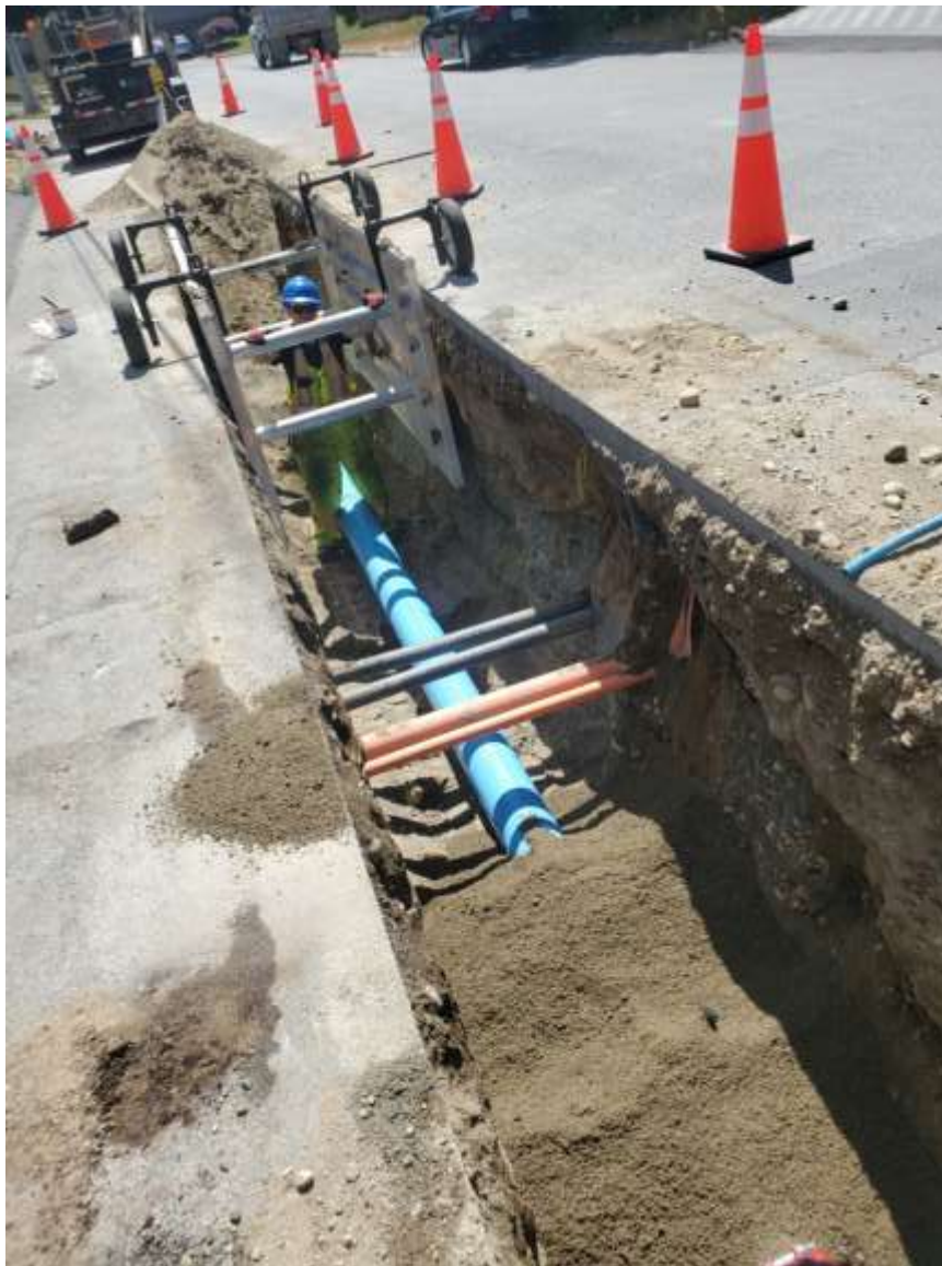
IMAGE | 2024 PIPE REPLACEMENT ALONG CARLA COURT - 200-MM BIONAX® PIPE WAS INSTALLED.
