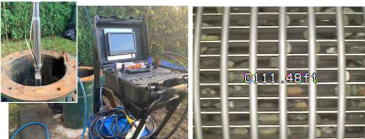
IMAGE | DOWNHOLE VIDEO INSPECTION EQUIPMENT (LEFT) AND VIDEO EXCERPT (RIGHT) - THE CAMERA IS DIRECTED TOWARDS THE WELL SCREEN AND GEOLOGICAL FORMATION.
