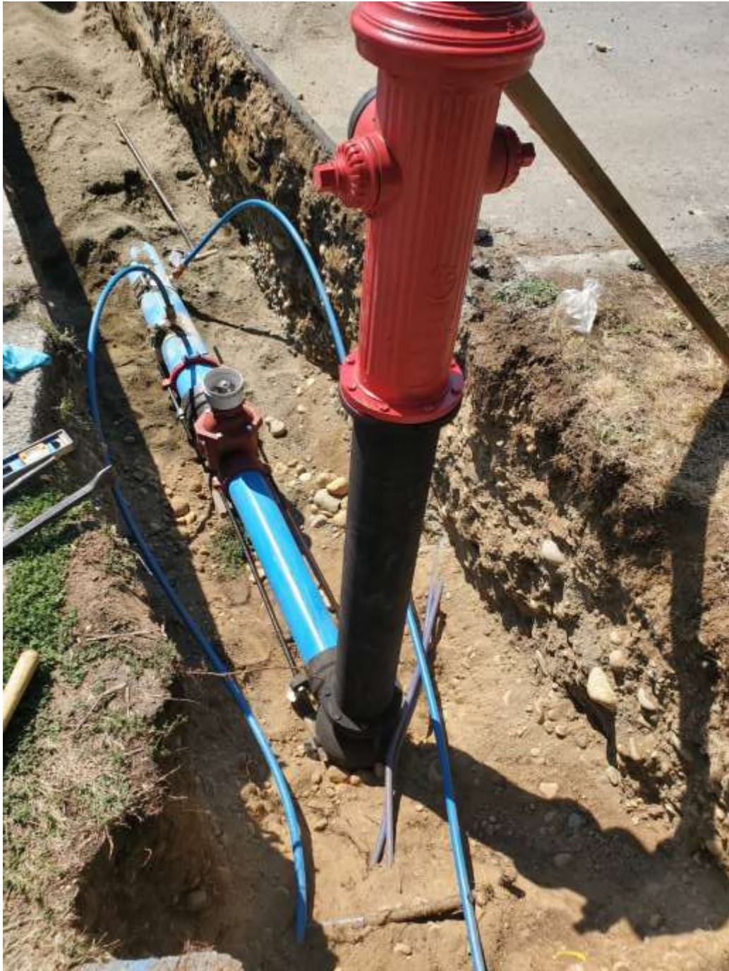
IMAGE | 2024 PIPE REPLACEMENT INCLUDED THE INSTALLATION OF 2 NEW FIRE HYDRANTS.
