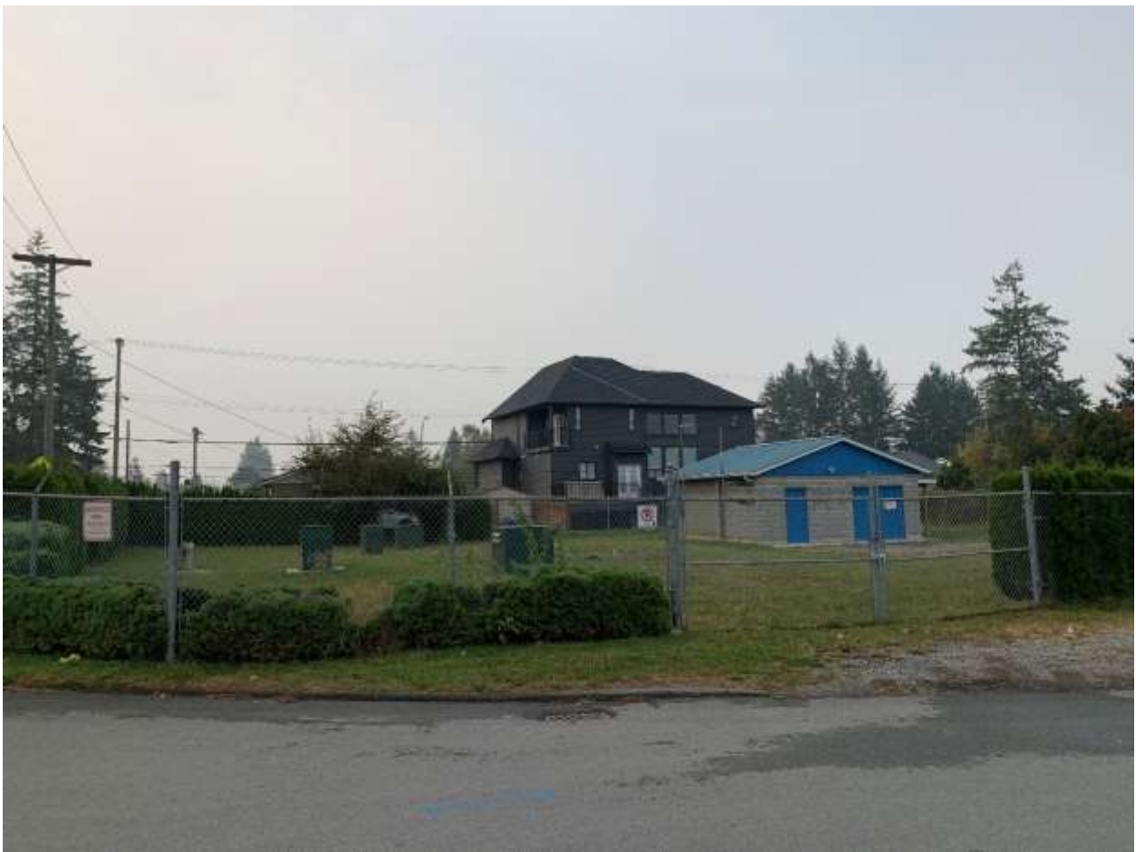
IMAGE | AUTUMN WELL FIELD: PUMP HOUSE AND RW 1-87/14.
