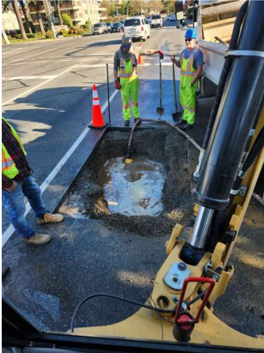
IMAGE | WATER MAIN LEAK REPAIR, ON CLEARBOOK ROAD, SOUTH OF OLD YALE ROAD.
