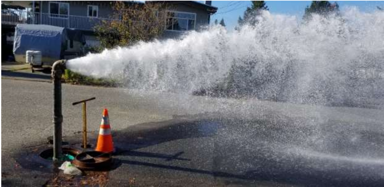
IMAGE | WATER SYSTEM FLUSHING IN PROGRESS.
